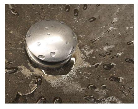
The drain was not the lowest point of the bathtub, hence the water was collecting just before the drain. This water will never drain out by itself - it either has to vaporize or be wiped off. It may just be a minor inconvenience, but if the defect is bigger it will more likely be frustrating.
