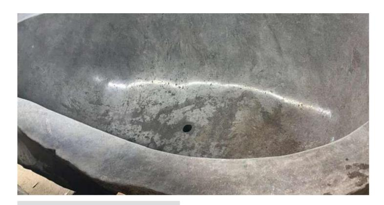
The middle of the the internal bottom was covered in transparent varnish (a type of paint that imitate the high polishing). It then started to come off leaving the surface rough and easy to soak water. Proper polishing takes time, therefore some suppliers skip this process by applying varnish. Through the miracle of time, however, the spell is broken and the true nature is always unravelled. Nothing is more reliable than the appropriate polishing.
