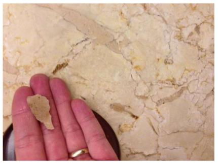
In this case, the inner surface of the marble bathtub was polished, but very badly. The users were at risk to be scratched by the uneven surface. Not to mention that everyone wants to get comfortable in such a bathtub. Covering the surface with glue or adhesive mortar will not do, the bathtub will still slowly soak water in the course of time.
